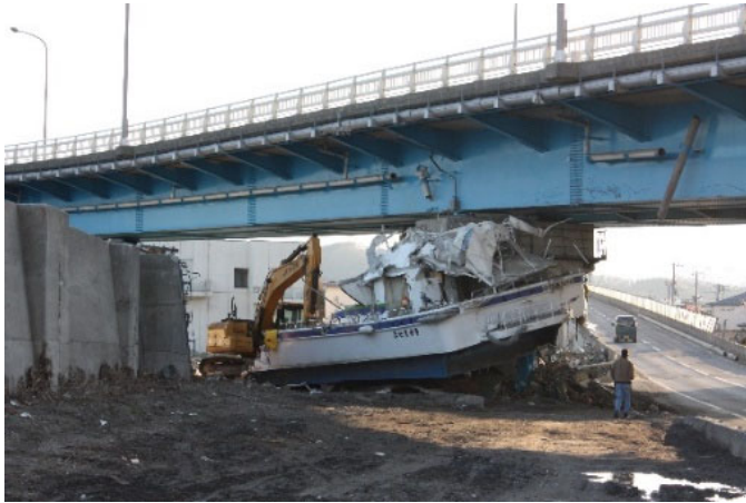
Figure 10 Ship collision damage (see online version for colours)
