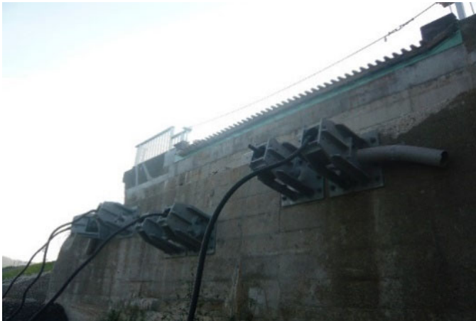
Figure 11 Tearing off of fall-off prevention devices (see online version for colours)
