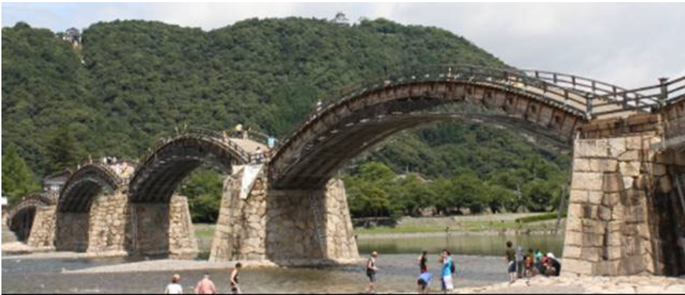
Figure 14 Kintaikyo Bridge as of 2009 (see online version for colours)
