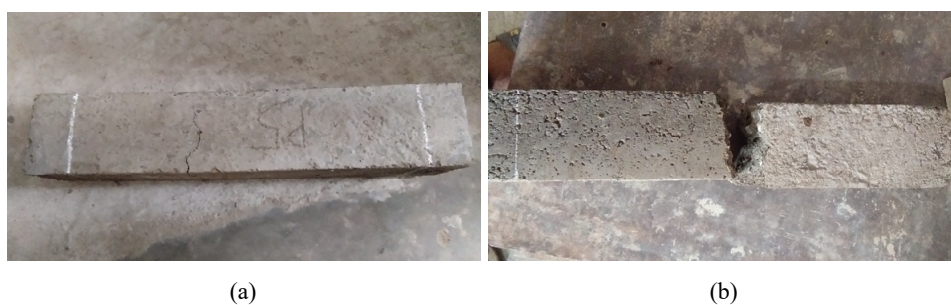
Figure 8 Crack propagation in the concrete beam after flexural strength test, (a) with (b) without using waste plastic as coarse aggregates (see online version for colours)
