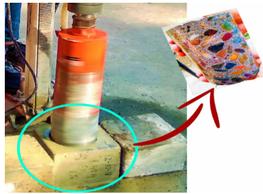
Figure 1 Core extraction from concrete cubes for control specimens (see online version for colours)
