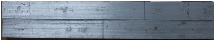
Figure 6 Beam with surface crack [scale 1:2] (see online version for colours)
