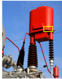
Figure 6 Comparison of defect detection results of low-voltage current transformer under electrification by different methods, (a) proposed method (b) method of Hu et al. (2021) (c) method of Luo and Xu (2021) (d) method of Wang et al. (2021a) (continued) (see online version for colours)
