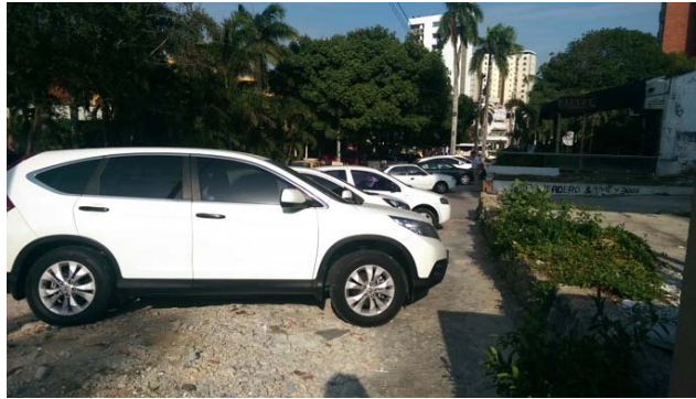
Figure 20 Cars parked on a footway that has been heavily damaged by parking (see online version for colours)
