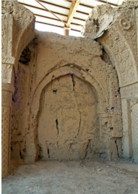
Figure 4 Internal view of South wall, central arch (see online version for colours)
