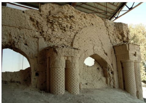
Figure 5 Internal view of north wall (see online version for colours)
