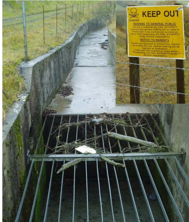
Figure 3 Blaenant land reclamation site, Wales: contour drain (with Juncus.sp ) showing erosional breaching of the contour bund (see online version for colours)
