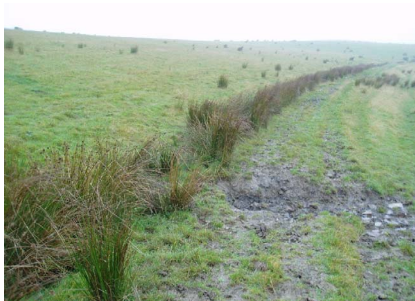
Figure 3 Blaenant land reclamation site, Wales: contour drain (with Juncus.sp ) showing erosional breaching of the contour bund (see online version for colours)
